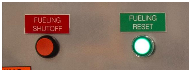
Figure 2-1 FUELING SHUTOFF AND FUELING RESET BUTTONS
