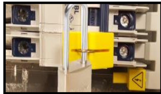
Figure 3-5 BREAKER LOCKED-OUT
