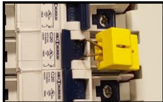
Figure 3-3 LOCKOUT ATTACHED
