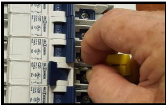
Figure 3-2 APPLYING LOCKOUT
