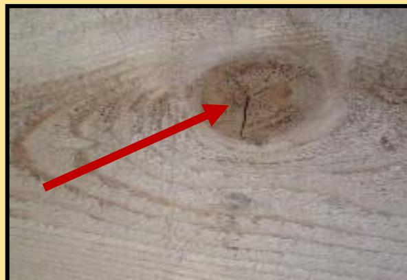
FIGURE 5 KNOTS ARE DARKER THAN THE WOOD; THEY MAY REQUIRE MULTIPLE COATS
