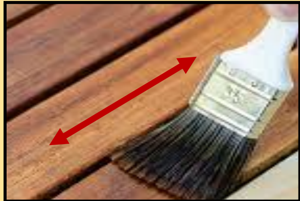
FIGURE 4 APPLY PRIMER WITH A BACK-AND-FORTH
